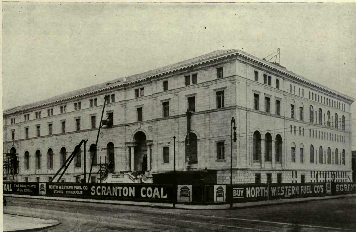
St. Paul Public Library, St. Paul, Minn. E. D. Litchfield, Architect All foundation work waterproofed with Truscon Waterproofing Paste, Concentrated.
